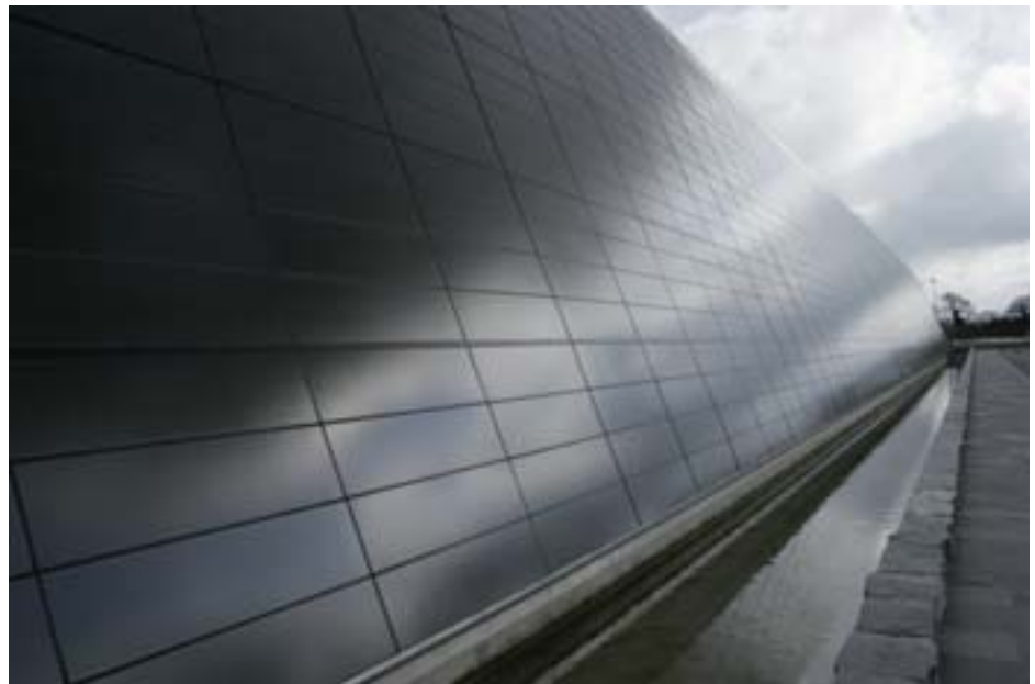
Figure 2. View of Solar Wall at OpTIC Technium.
